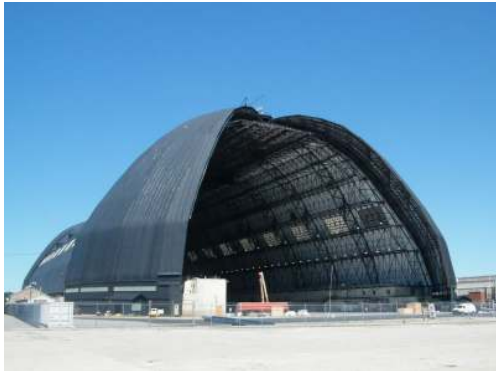
Photo: Conring Automation Services
