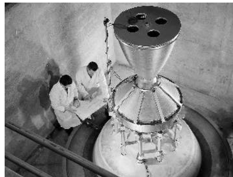
Technicians manufacture a nozzle for the Kiwi B-1-B nuclear rocket engine as part of the NERVA programme. Photo: NASA / GRC
